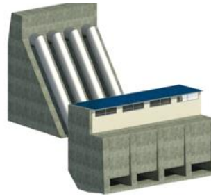
Vertical Francis turbine and water intake
